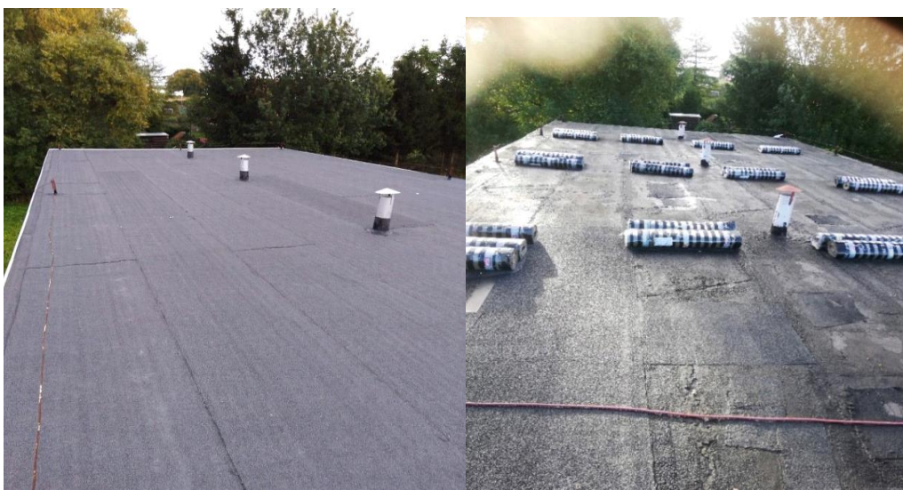
Remont dachu SUW Wandajny
