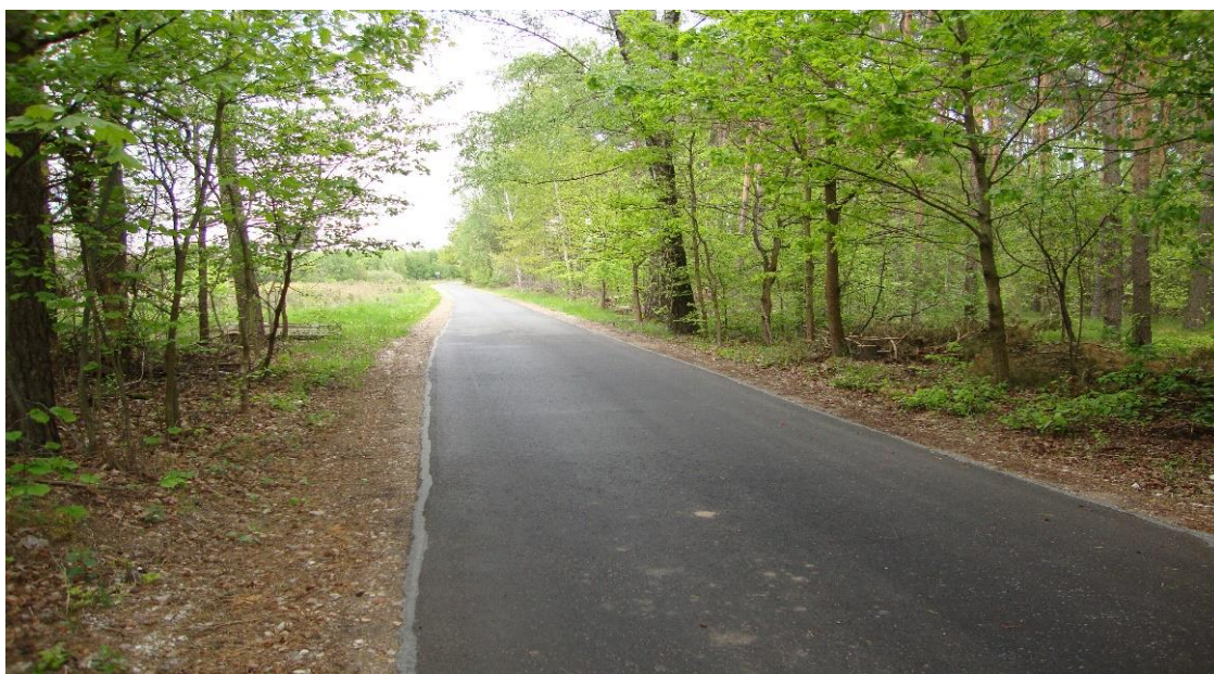
Droga gminna w Rydzewo.
